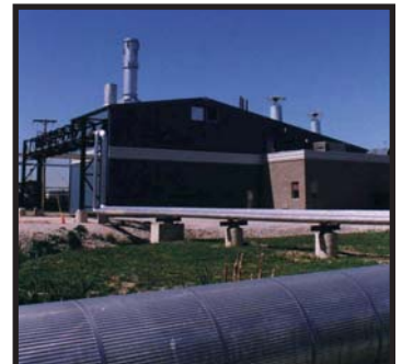
The 6000-square foot cogeneration building is set well back from the main production area to permit future expansion. The large metal pipe carries steam and hot water back to the processing floor.
