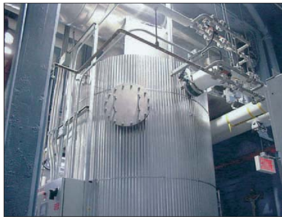
Figure 1 (left): New energy-efficient boilers; (top right) Collège Jean-de-Brébeuf; (bottom right) condensing stack economizer.
