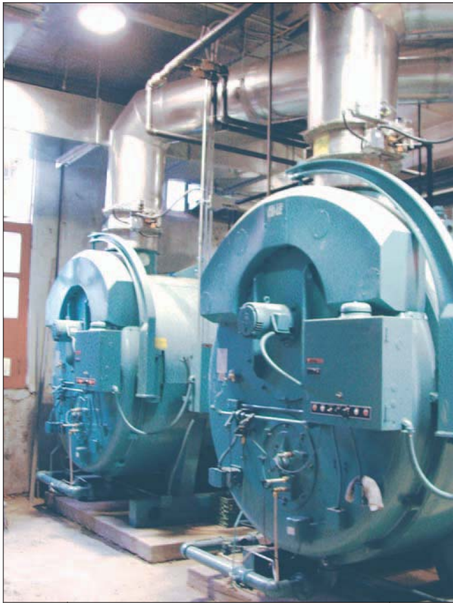
Figure 1 (left): New energy-efficient boilers; (top right) Collège Jean-de-Brébeuf; (bottom right) condensing stack economizer.
